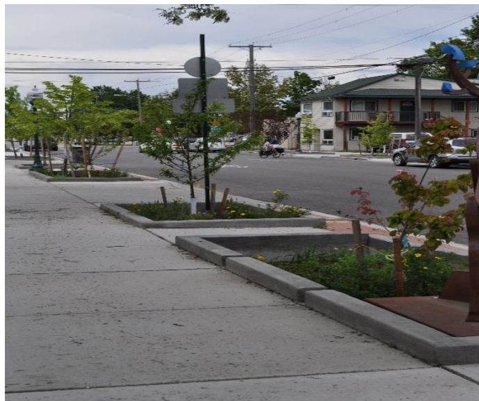
Sandpoint: Street Reconstruction
