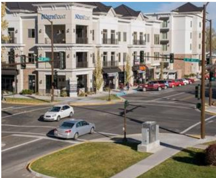
Rexburg: Traffic Signal to Improve Safety
