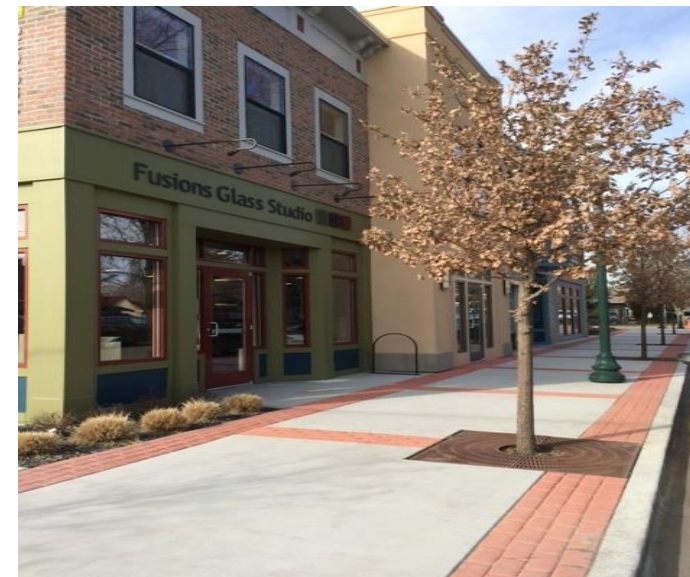
Eagle: Right-of-Way Improvements
