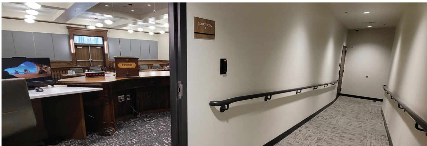
A ramp in the new Nez Perce County Courthouse, showing the more accessible building and updated facility.
