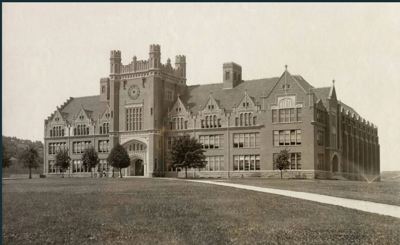
Administration Building, University of Idaho, 1912. Photo credit: University of Idaho Campus Photographs, [University of Idaho Library Special Collections and Archives, PG1_52 10].
